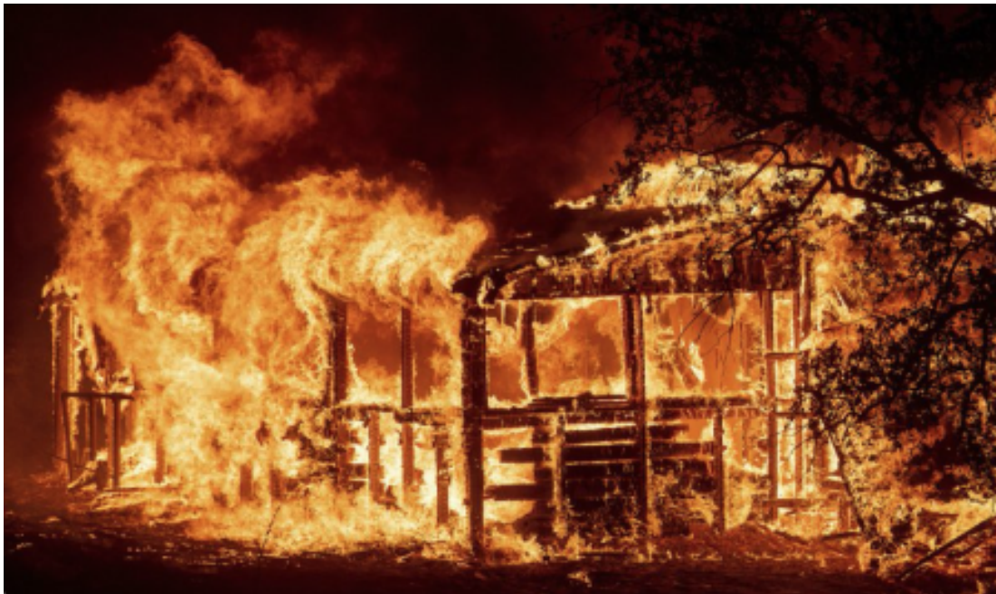
A fully engulfed structure along HWY 299 near Redding California. Photo credit: AP/Noah Berger
